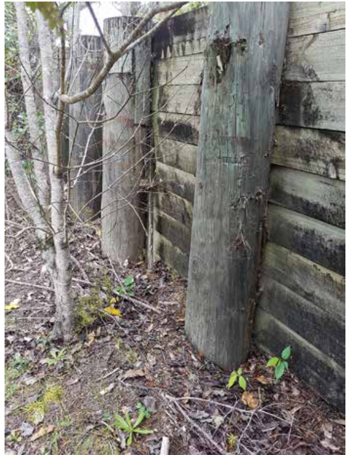
Timber cantilever retaining wall
