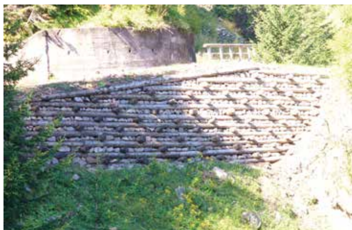
Treated timber crib as retaining wall of forest road fill slope. Never use untreated radiata logs as they are not durable
