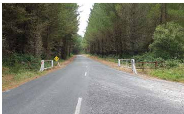
A sealed forest arterial road
