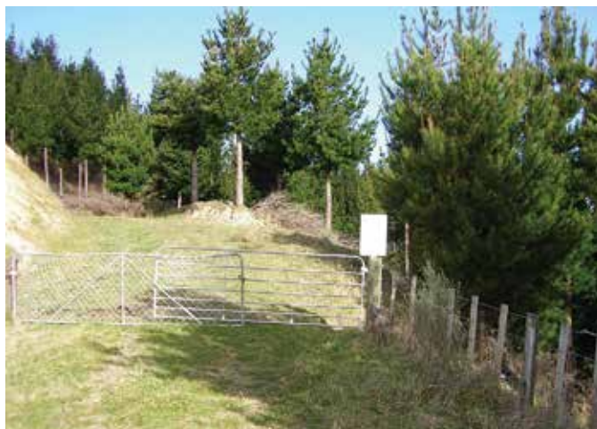
A typical establishment track, gated to restrict access and grassed to eliminate on-going erosion
