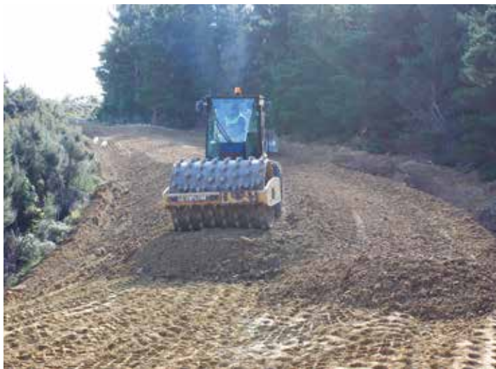
Compaction needs to be done in layers
