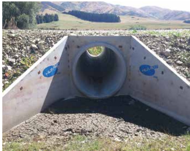
Examples of smooth-bore concrete pipe culverts with and without wingwalls. The photo below demonstrates the potential issue of fish passage, due to high water velocity
