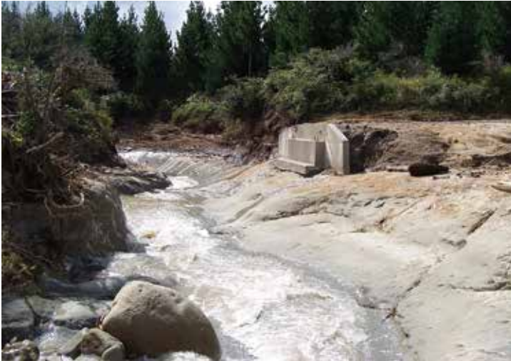
Left: Bridges can become part of a debris flow even in a well-sited location. Make sure the bridge soffit is at least 1 m above a 2% AEP event. Right: The replacement is a metre higher
