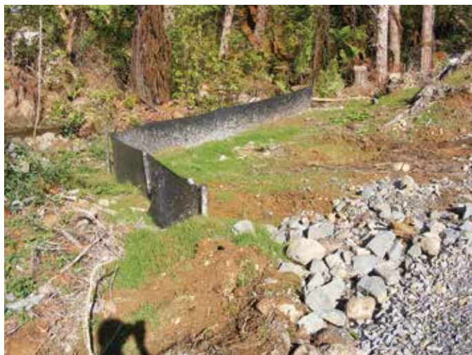
Two well-constructed applications for sediment fences
