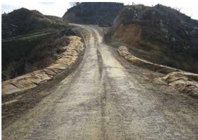
Left: Well-compacted berms were used to protect a large fill slope by directing water away from the more vulnerable earthworks. Water has been directed to cut-outs and flumes on either side of the fill. Right: This large fill is showing failure, despite having cut-outs and flumes, and will lead to environmental and access issues unless modified. The berms are too small, and the low point of the road is in the middle of a large fill slope, rather at one end where the water can be more easily directed to original ground
