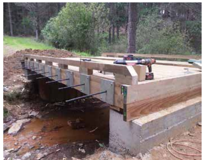
An option to concrete and steel – a New Zealand designed composite post-tensioned treated wood composite bridge
