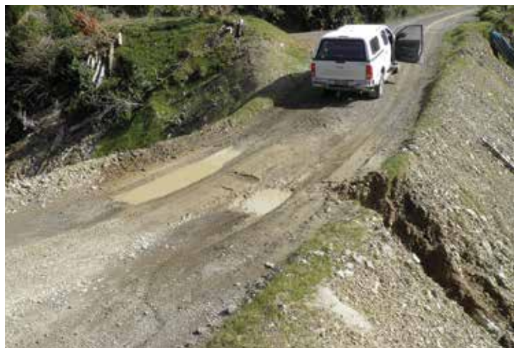
Left: Well-compacted berms were used to protect a large fill slope by directing water away from the more vulnerable earthworks. Water has been directed to cut-outs and flumes on either side of the fill. Right: This large fill is showing failure, despite having cut-outs and flumes, and will lead to environmental and access issues unless modified. The berms are too small, and the low point of the road is in the middle of a large fill slope, rather at one end where the water can be more easily directed to original ground
