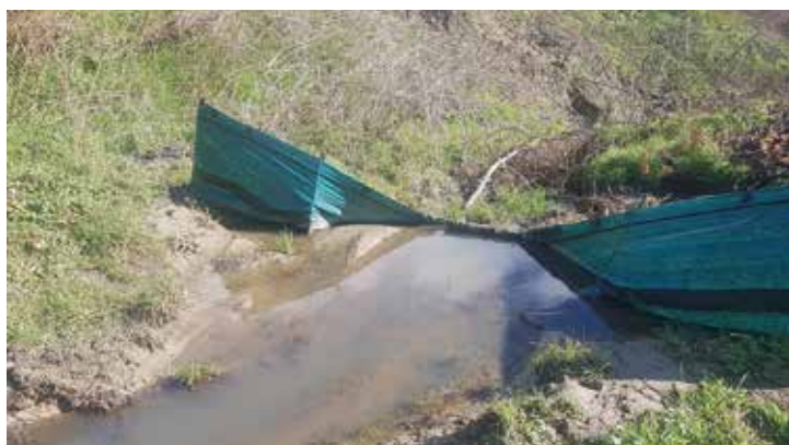
Left: Sediment fences are not designed for watercourses. They fill rapidly, divert flow, or fail. Right: This fence is inadequate. The lower edge has not been buried properly, so has blown out. The fence is not wide enough, and there are no wings so stormwater flow would have bypassed it. Also, it is too close to the waterway immediately behind it
