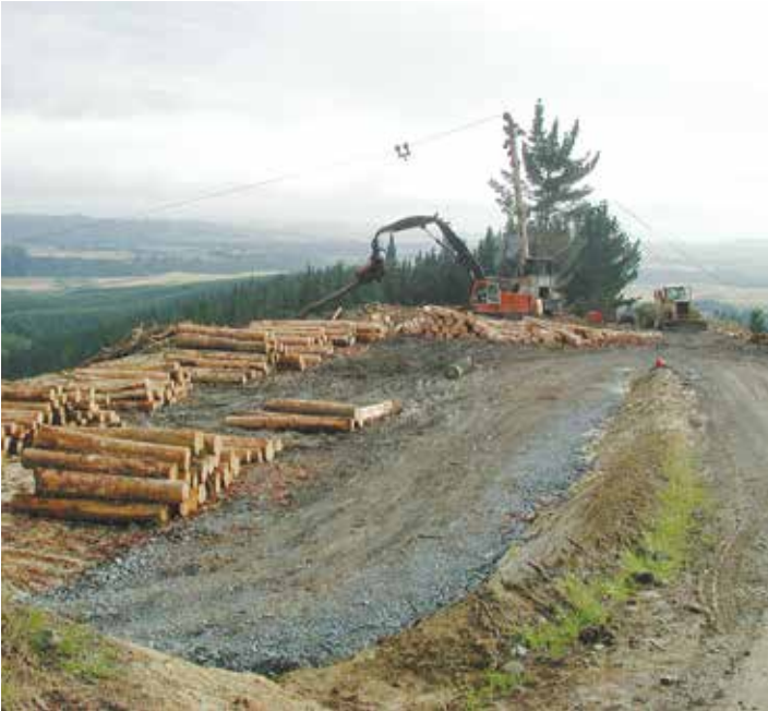
Spur road landing
