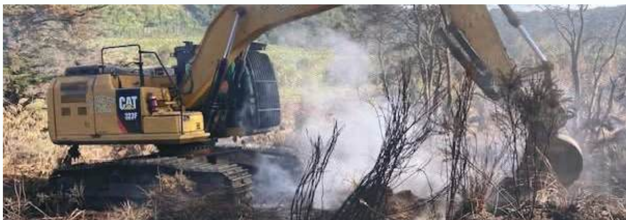
↑ Image by Peter Houston – Digger Opening Up Hot Spots
