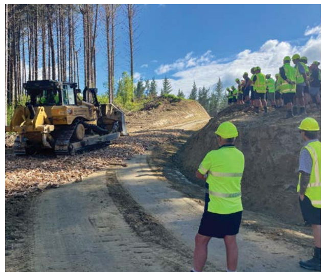
↑ Foresters in Pan Pac's Mohaka Forest watching a trial turning wood residues into roading material. Image; Pan Pac Forest Products Ltd
