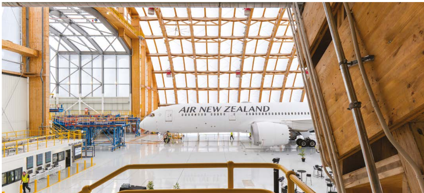
↑ Hangar 4 is expected to store carbon for decades, likely beyond 60 years. Its sustainability performance earned it a 6 Green Star certification. Photo; Studio Pacific
