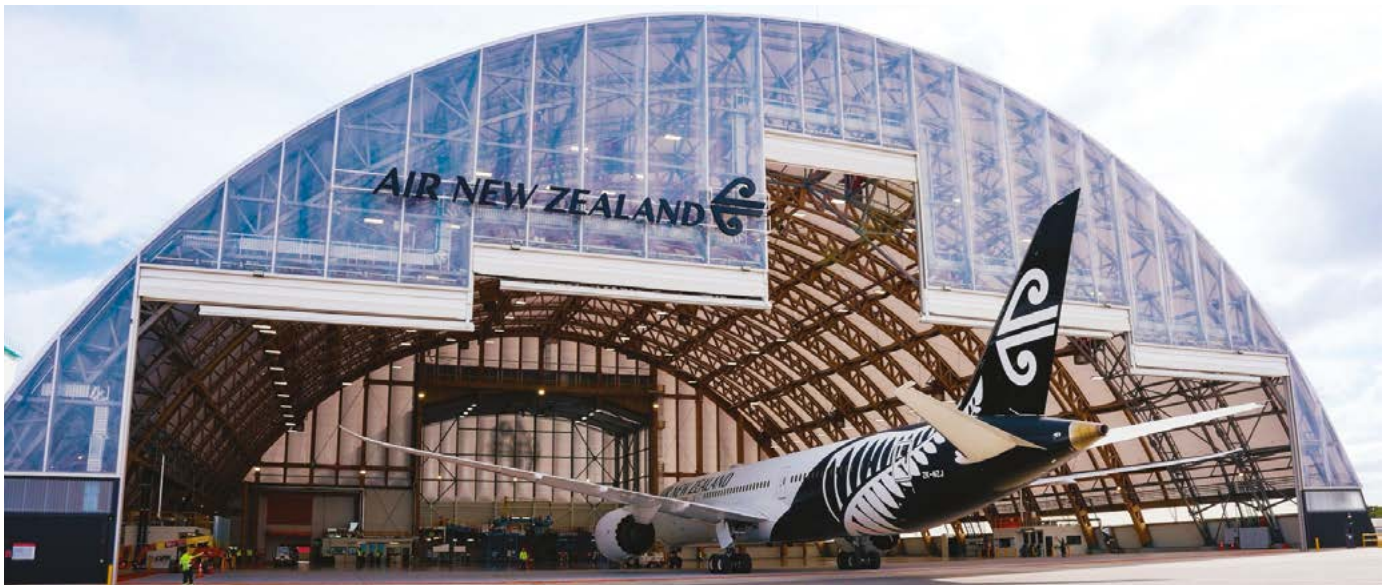
↑ Air New Zealand's new aircraft hangar features the largest single-span engineered timber arch in a Southern Hemisphere hangar. Photo; Air New Zealand
