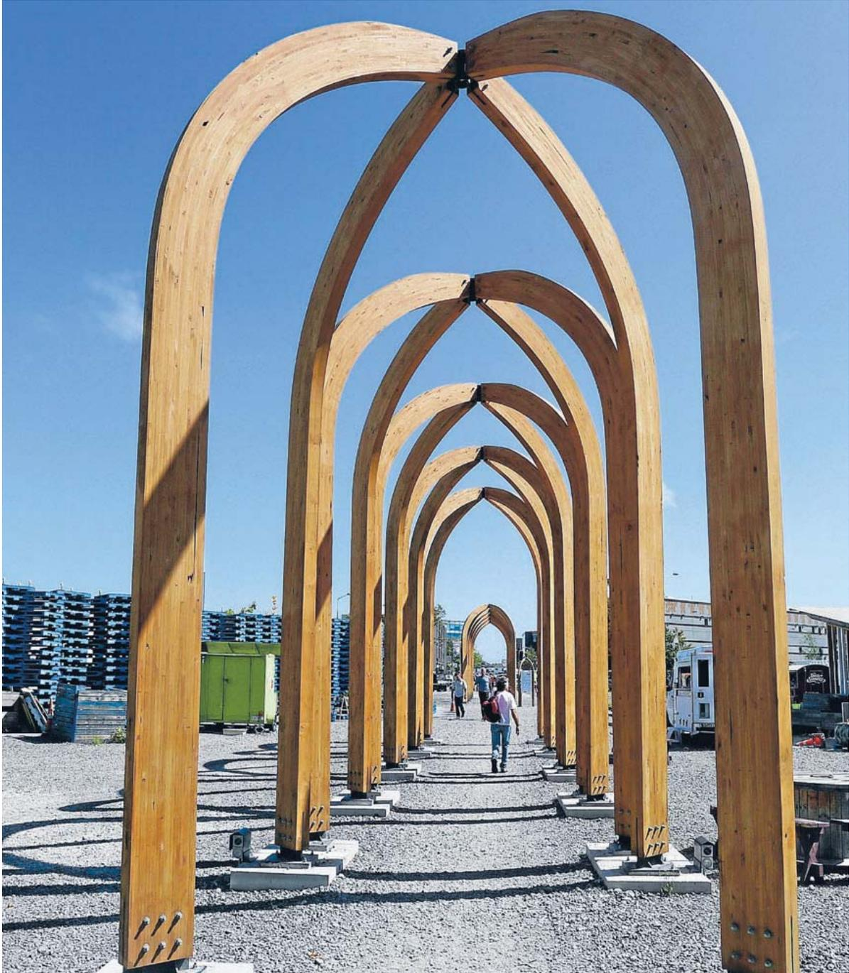
**Wood on show:** The Arcades, on the old Crowne Plaza site in central Christchurch, is a 6m high installation made from Glulam engineered timber.
