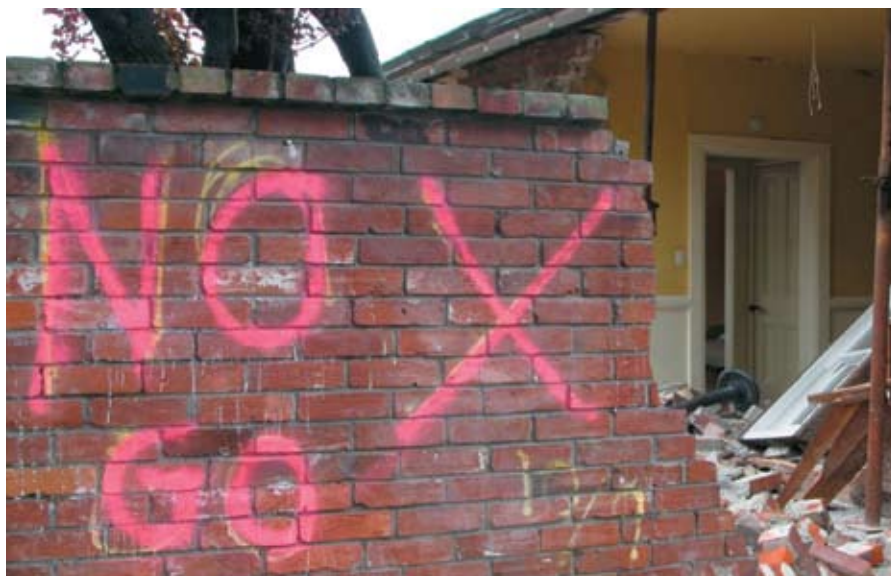
The rebuilds of Christchurch and Japan will do much to trigger renewed demand for lumber and processed wood products. Image: www.raw.co.nz
