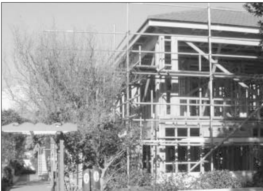
Untreated Radiata and Douglas fir are excellent framing timbers in most situations
